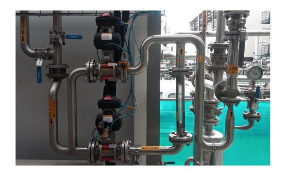
H<sub>2</sub> dilution in normal vent done using N<sub>2</sub> ejector. High nitrogene flow produces higher vacum in Venturi system.
