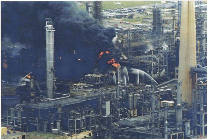
View from south west showing fire at flare drum (photograph courtesy of the Western Mail and Echo Ltd)
