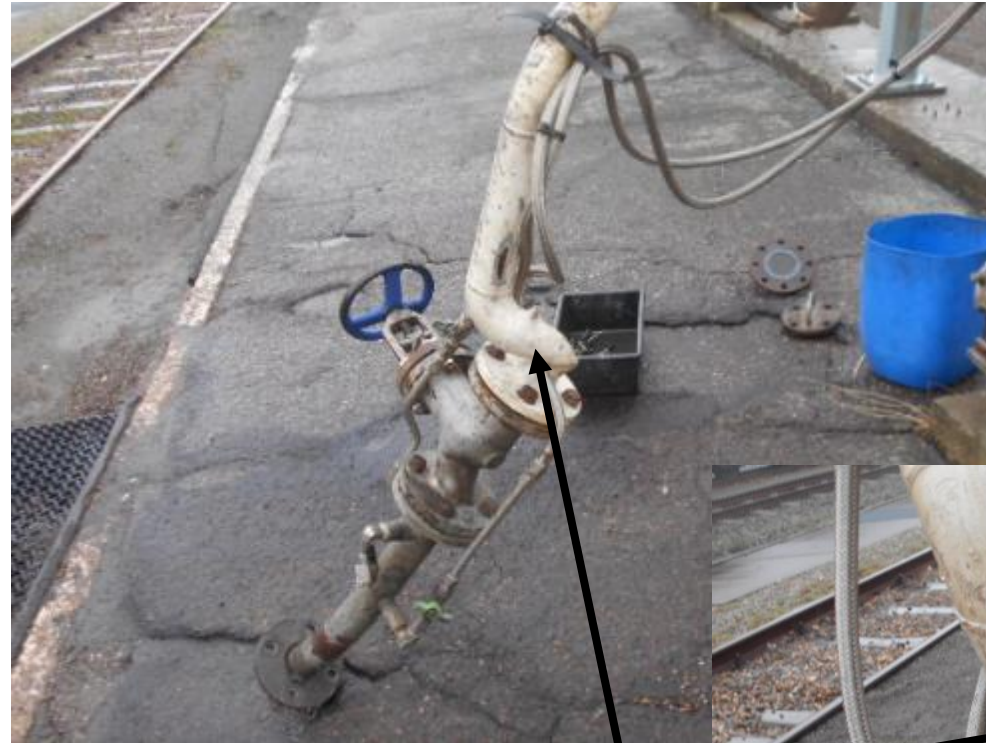
Loading arms gas and liquid phase severely damaged but not leaking
