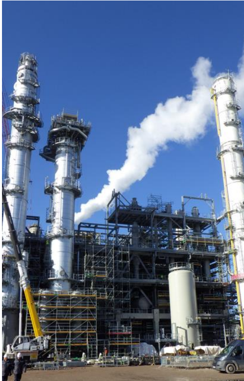
Erection of scaffold
