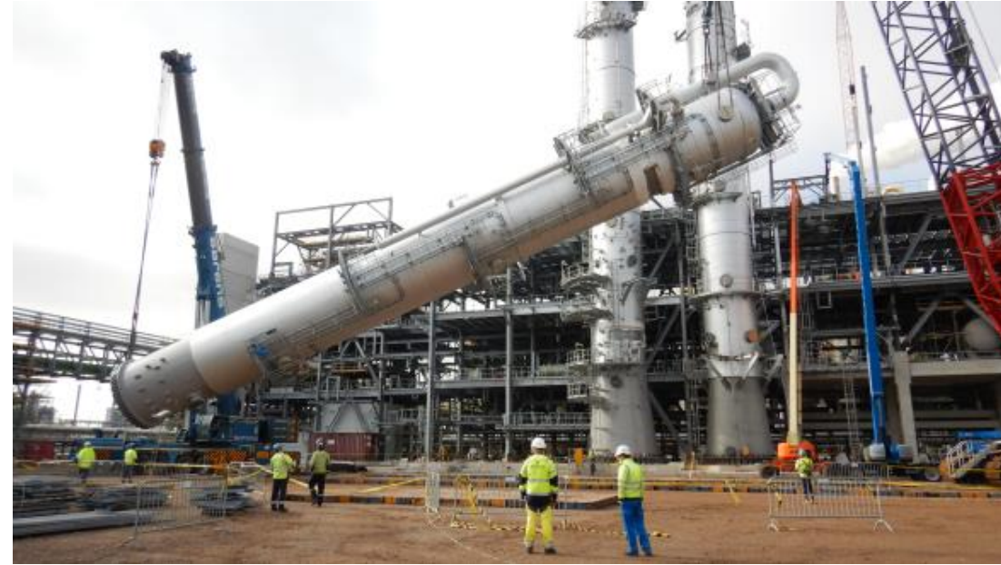
Lifting CO2 Absorber
