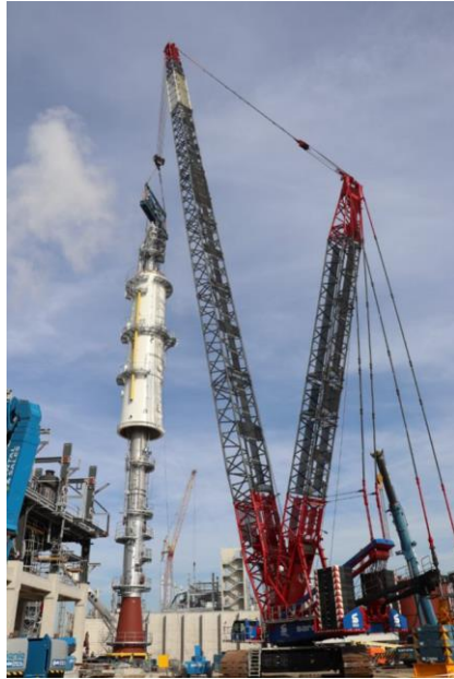
Installation PEO column and casing
